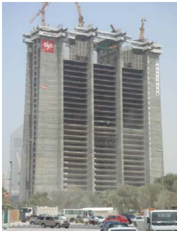
Figure 9. Index Building under Construction (Foster + Partners, 2007)
