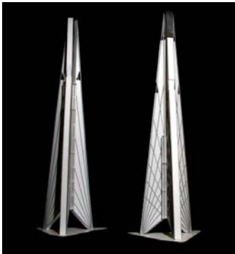
Figure 19. Add reverse Fan columns (Foster + Partners, 2005)
